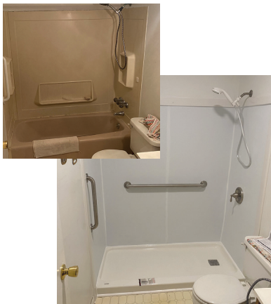
New shower stall before/after
