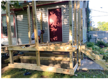
New entrance deck under construction
